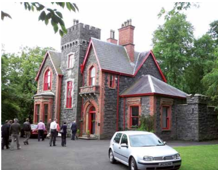
▲ On the road to the reception building of the Patton Group
